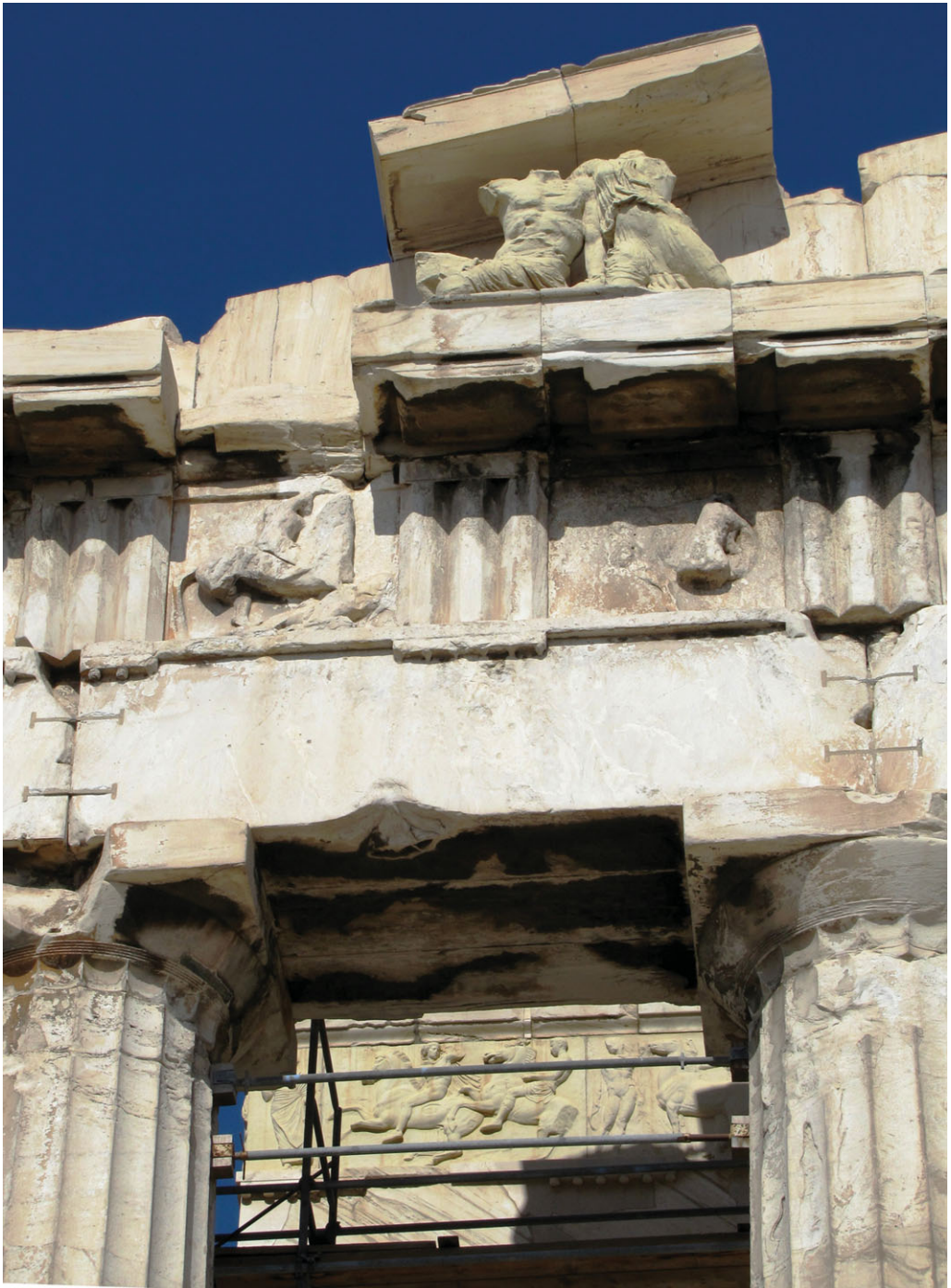
Figure 2. The west side of the Parthenon, during its restoration in 2010: all sculpted decoration (pediment, metopes and frieze) is modern.
